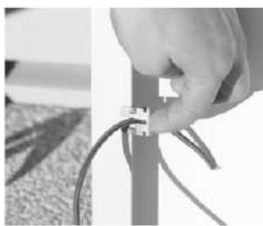
1 Position grounding clip with electrical cable inserted in it and the bottom of the part outside the frame
