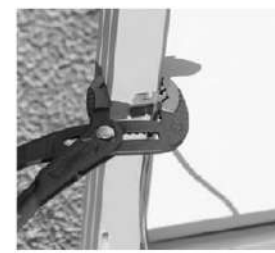
3 Grip up to the stops of the clip are against the frame
