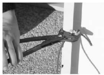
2 Place the plier by gripping the clip with the external jaw and internal jaw set on external face of the module frame
